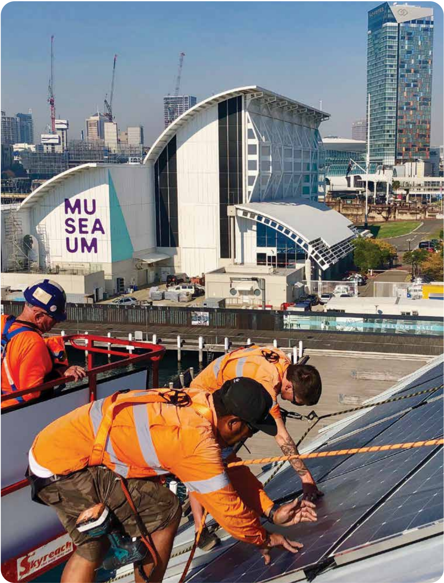
Technicians install some of the 812 solar panels on the roof of the Wharf 7 building. Image Rene Hernandez/ANMM
