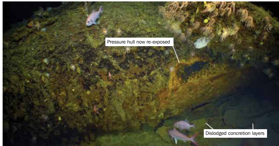
Figure 47 – Example of concrete delamination under foreplane. Image courtesy of Paul G Allen, Find AE1, Australian National Maritime Museum and Curtin University. © Navigea Ltd
